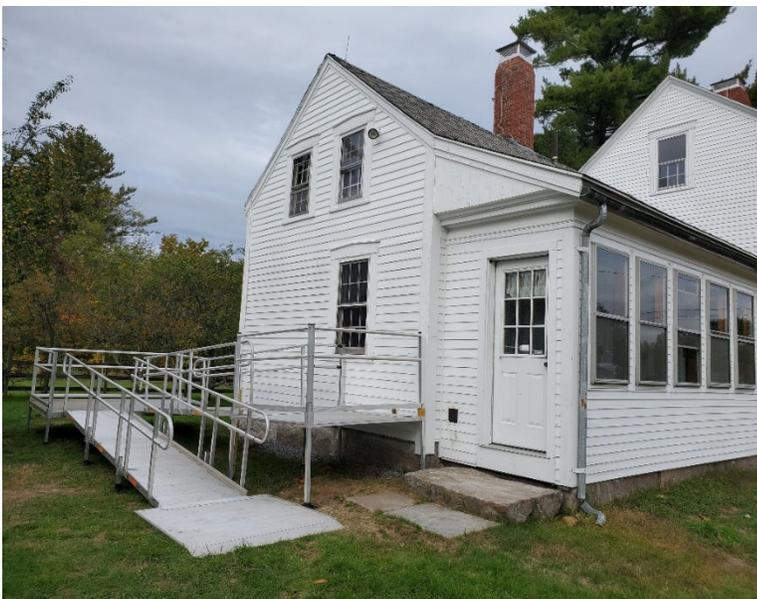
This ramp had all the hand railings included, and very roomy landings. The self-leveling design makes for greater ease of assembly.
